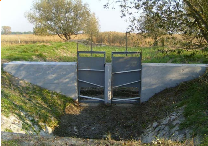
Figure 1: Water retention works
