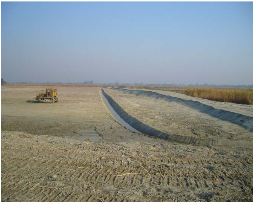
Figure 2: Water retention reservoir
